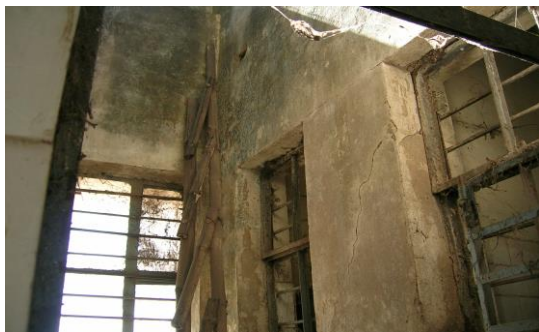
Fig. 4: Fungal spores at unattended damp areas
