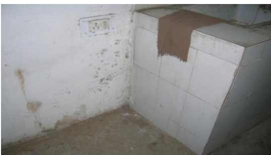
Fig. 6: Below the sink moist area showing spores of fungi and mold
