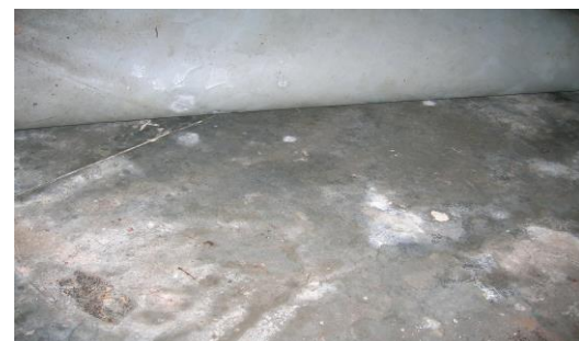
Fig. 2: Growth of mold and fungal spores below the carpet
